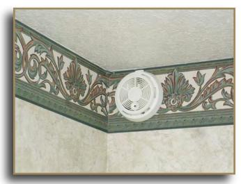
air space here where smoke and other combustion products may not be able to reach the detection chamber.
